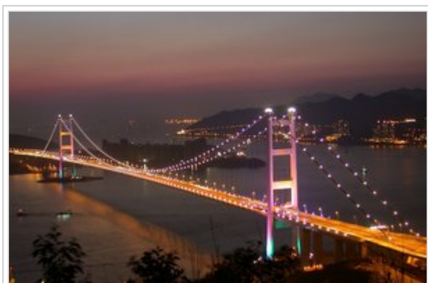
Tsing Ma Bridge, Hong Kong
