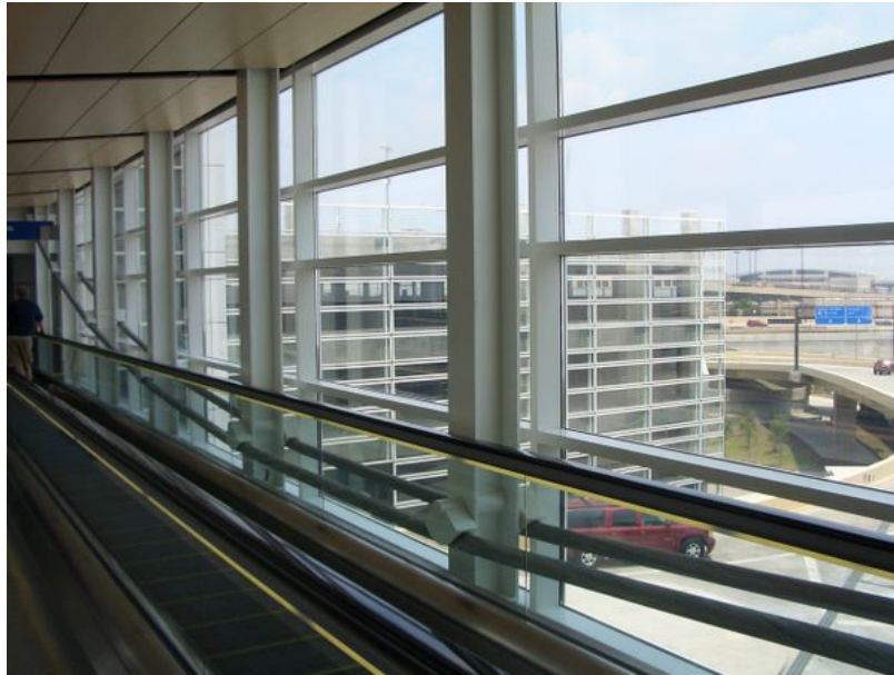
Cable-suspended footbridge at Dallas Fort Worth Airport Terminal D
