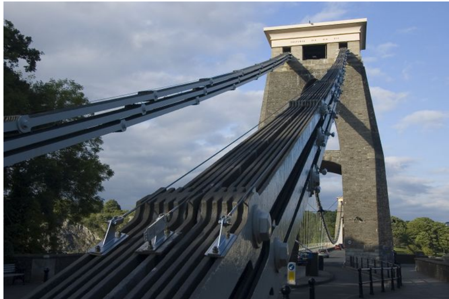
Eyebar chain cables of Clifton Suspension Bridge
