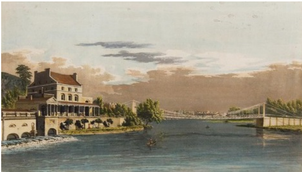
Wire Bridge at Fairmount (1842, replaced 1874).
